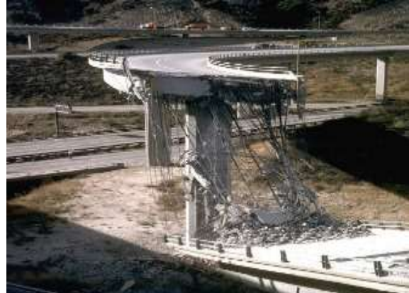
Fig. 5 A superstructure failure
